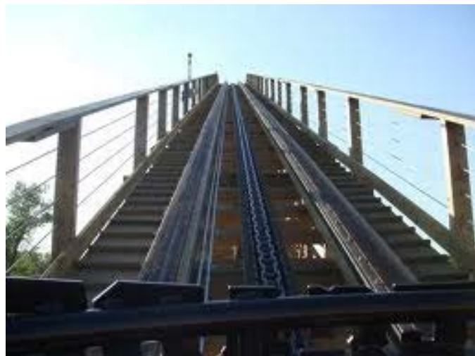
Figure 5: Chain Lift
