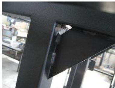
Figure 10 Cooling Tower Frame
